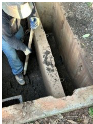
Stormwater Bunker Cleanout 8+ inches of mud and muck!
